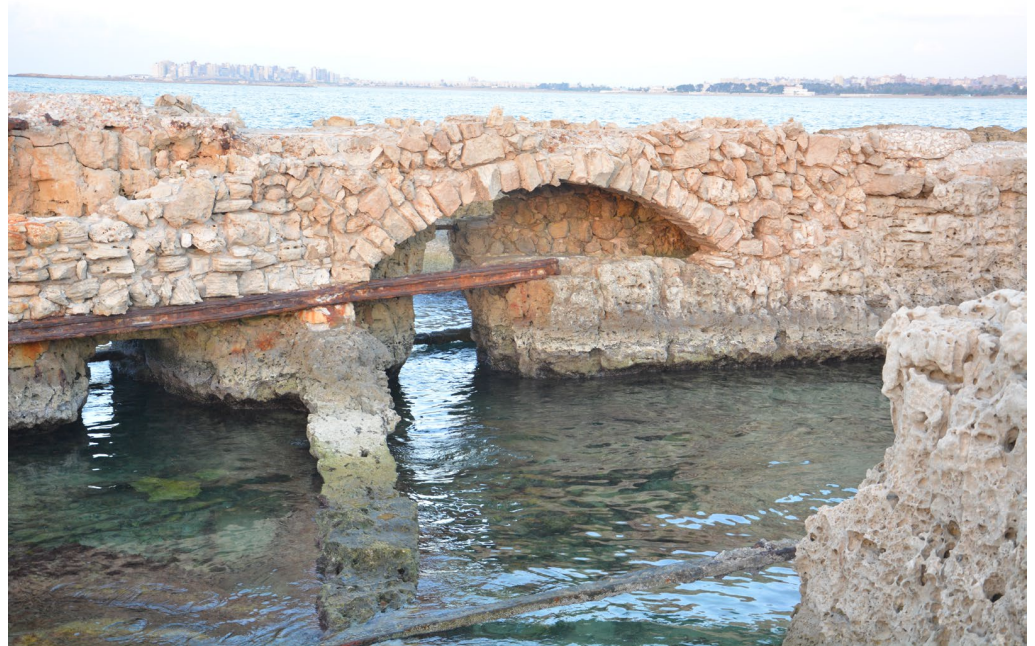
Figure 3. Arching wall at the Montazah fish tank of Alexandria, Egypt, along with the channels that distributed water within the tank, ensuring its adequate circulation within the construction.
