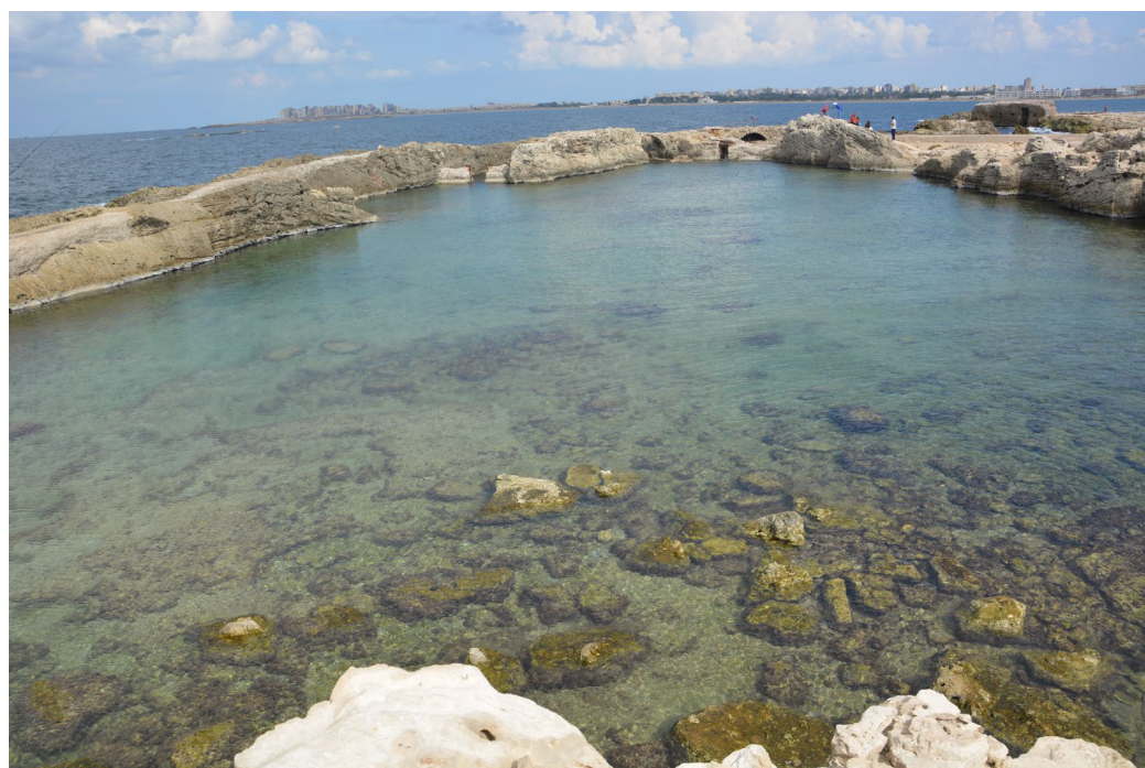
Figure 12. The western part of the Montazah fish tank in Alexandria, Egypt.
