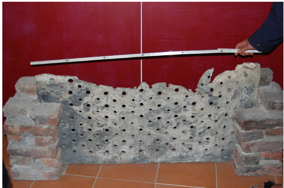
Figure 6. Sluice gate (cataracta) from the Grottafce fish tank, Italy, presently at the Santa Marinella Museum.
