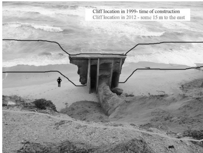
Fig. 12 - A sewer outlet in Ashkelon North, demonstrating the cliff retreat of 1 m yearly. The black lines depicts the location of the coastal cliff in 1999, the bright line indicates the present cliff edge (E.G.).
