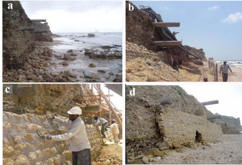
Fig. 14 - Ashkelon sea wall under reconstruction works: a) before works, b, c) a protective layer is being built on the wall face, d) the protective layer underwent erosion by the storm waves (E.G.).
