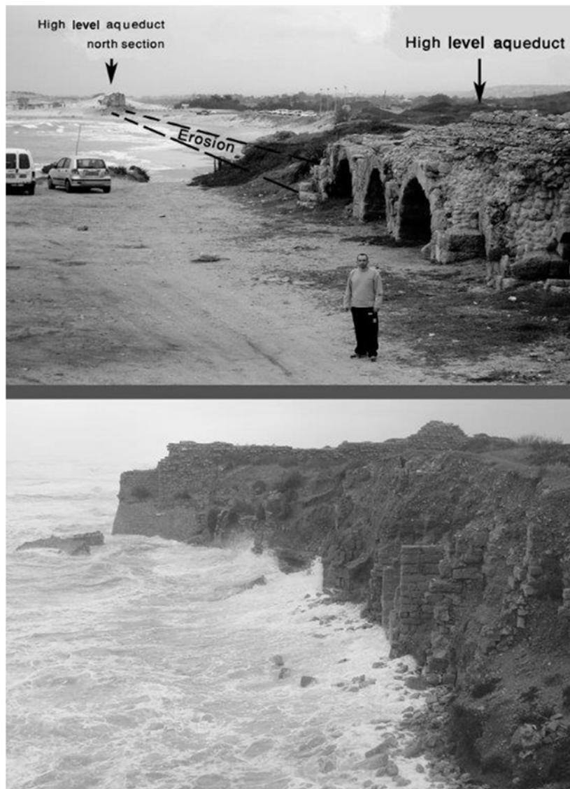
Fig. 5 - Top: the Roman high level aqueduct in Caesarea- a 500 m section of the aqueduct was eroded in the past; Bottom: the Byzantine city ruins undergoing marine erosion (E.G.).
