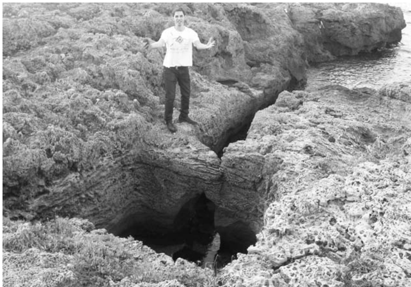
Fig. 10. Sea water well used as a pumping station for the production of salt, Habonim, Carmel coast (EG)
