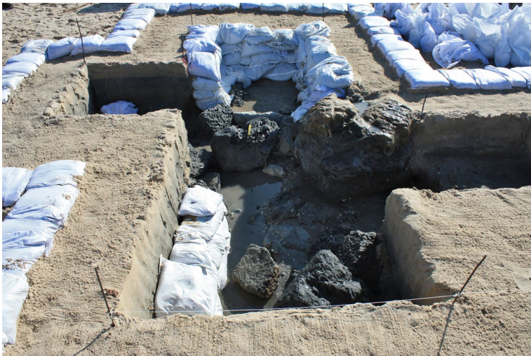
Fig. 8 Final photo of the excavation of Bollard DN44, facing south
