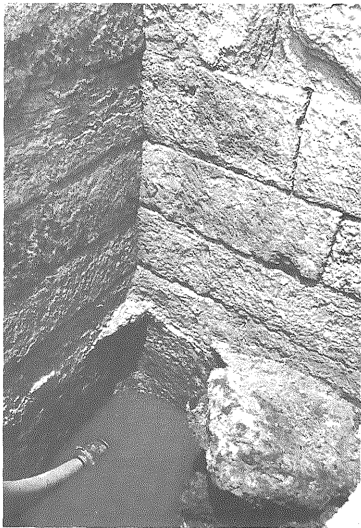
Photo 9.74. The northwestern side of the rectangular well; note the encrusted layer, representing the recent elevation of the ground water.
