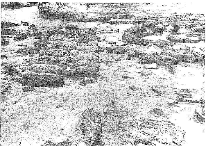
Photo 9.28. Ashlar sea wall on top of earlier rock-cut channel on the northwestern side of the industrial complex, looking north.
