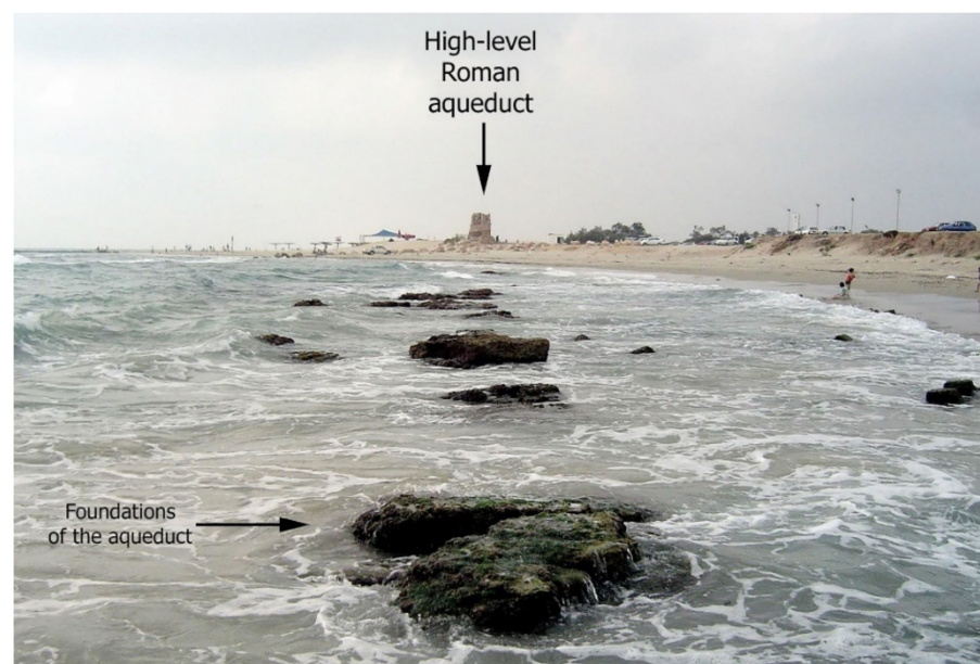
Figure 13. The remains of the aqueduct foundations after undergoing erosion in the sea and in situ on the coast, looking north (for location see Figure 6g).
