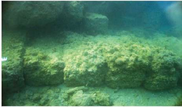
[16] Ashlars set as headers in a jetty on the southern bank of the bay, west of Kibbutz Sedot Yam (photography: Ehud Galili).
