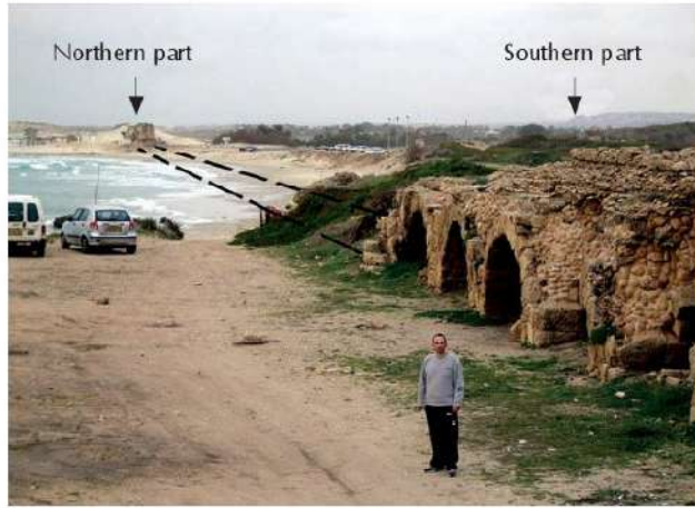
[17] Ruined portion of the high-level aqueduct on the shoreline of the northern anchorage, and foundations of the aqueduct, now submerged (photography: Ehud Galili).
