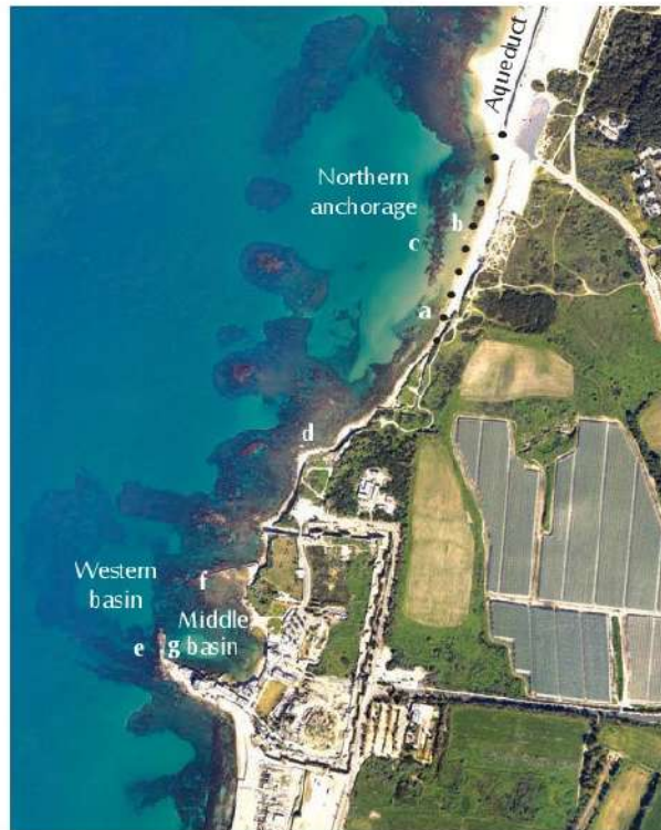
[20] Caesarea harbor, aerial view to the north: the submerged western basin; the northern basin; and the northern anchorage, where a portion of the aqueduct was apparently destroyed by the construction of the harbor (marked with black dots) (photography: courtesy of the Survey of Israel).
