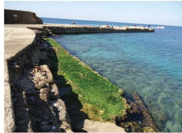
[18] Jetty built of headers in the middle basin, remains of the Herodian port (photography: Ehud Galili).
