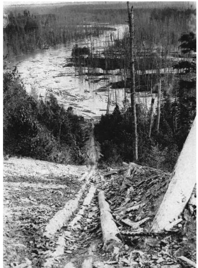
Fig. 12: Slides for facilitating the transport of logs into the river ahead of the drive. Source unknown. Available at http://www.geo.msu.edu/geogmich/river-logging.html
