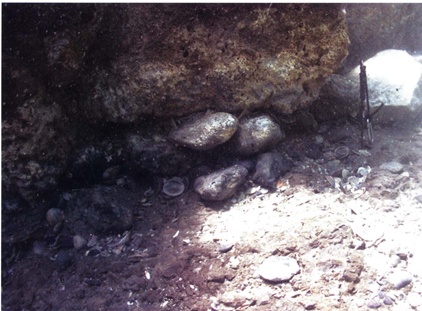
Pebbles placed under the eastern mole foundation provided for stability. Photo by S. Breitstein.
