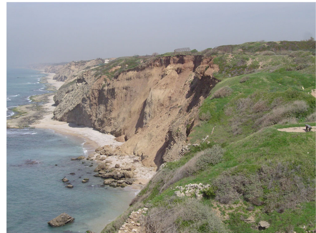
Fig. 5 Fresh landslide on the Apollonia coastal cliff (DZ)
