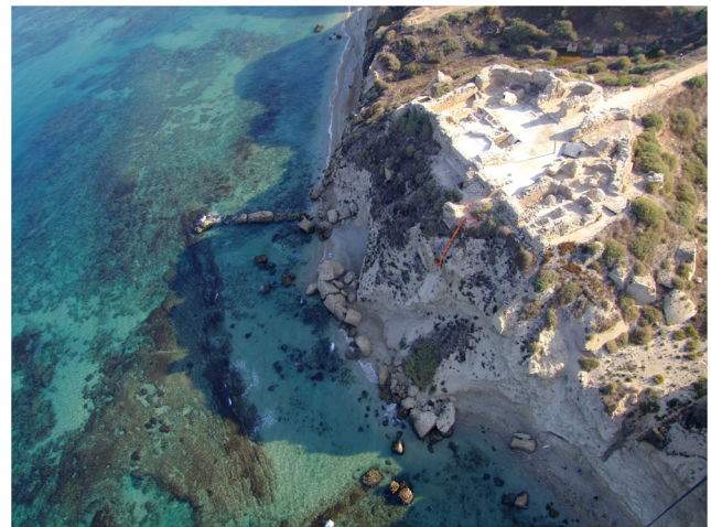
Fig. 8 The trapezoidal structure at the sea front of Apollonia (O. Tal, D. Mirkin)
