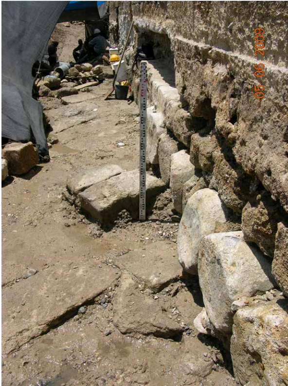
Figure 7. North-south view of the Hellenistic docking platform (Area C) after removal of the British Mandate reinforcement of cement beam and sacks. The exposed wall foundations are comprised of marble, granite, and kurkar columns placed directly on the Hellenistic quay (Photo: J. Sharvit).
