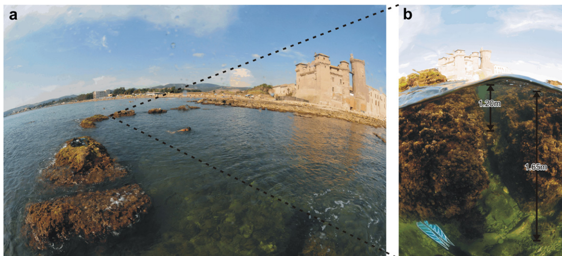
Fig. 7. a) Perimeter walls of the Pyrgi fishtank; b) particulars and measurements of the channel in the northern part of the fishtank.
