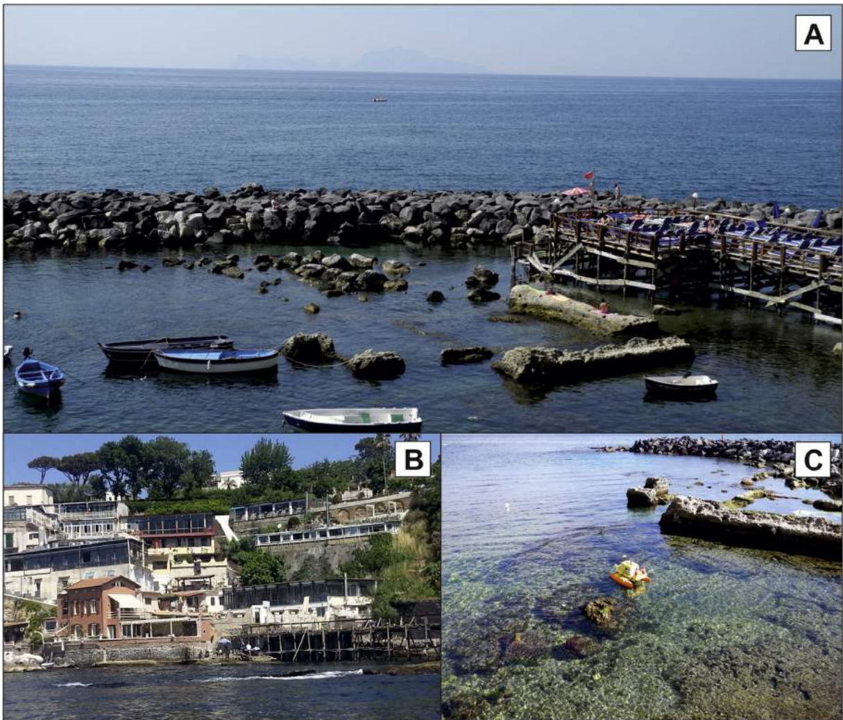
Fig. 9. A) panoramic view of the Marechiaro port close to Palazzo degli Spiriti; B) Submerged breakwater of the port; C) rests of the small villa near to the port.
