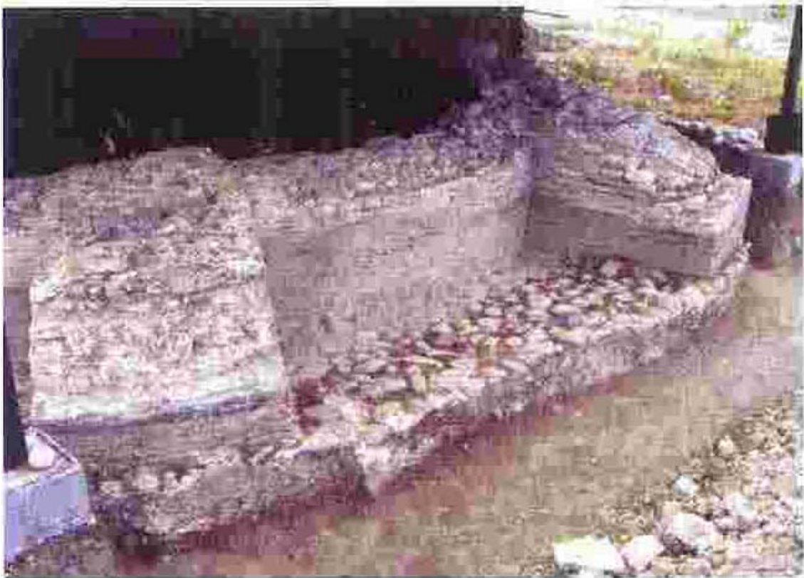
4.37. Buttresses of Room A. 213
