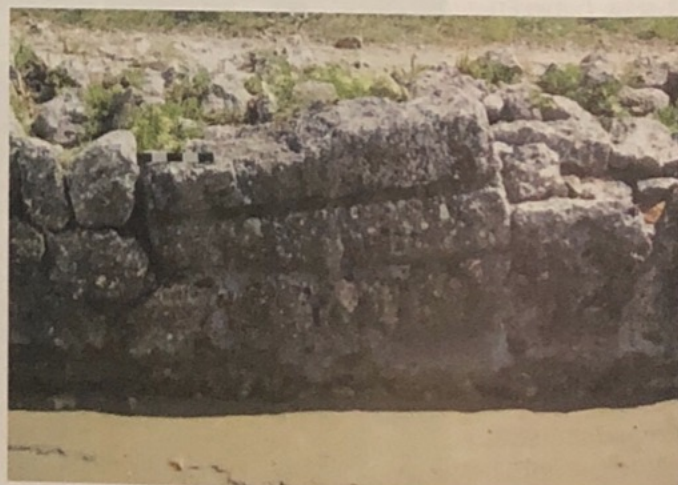
Fig. 11: One of the blocks for the cataractae , reused in the modern walls.
