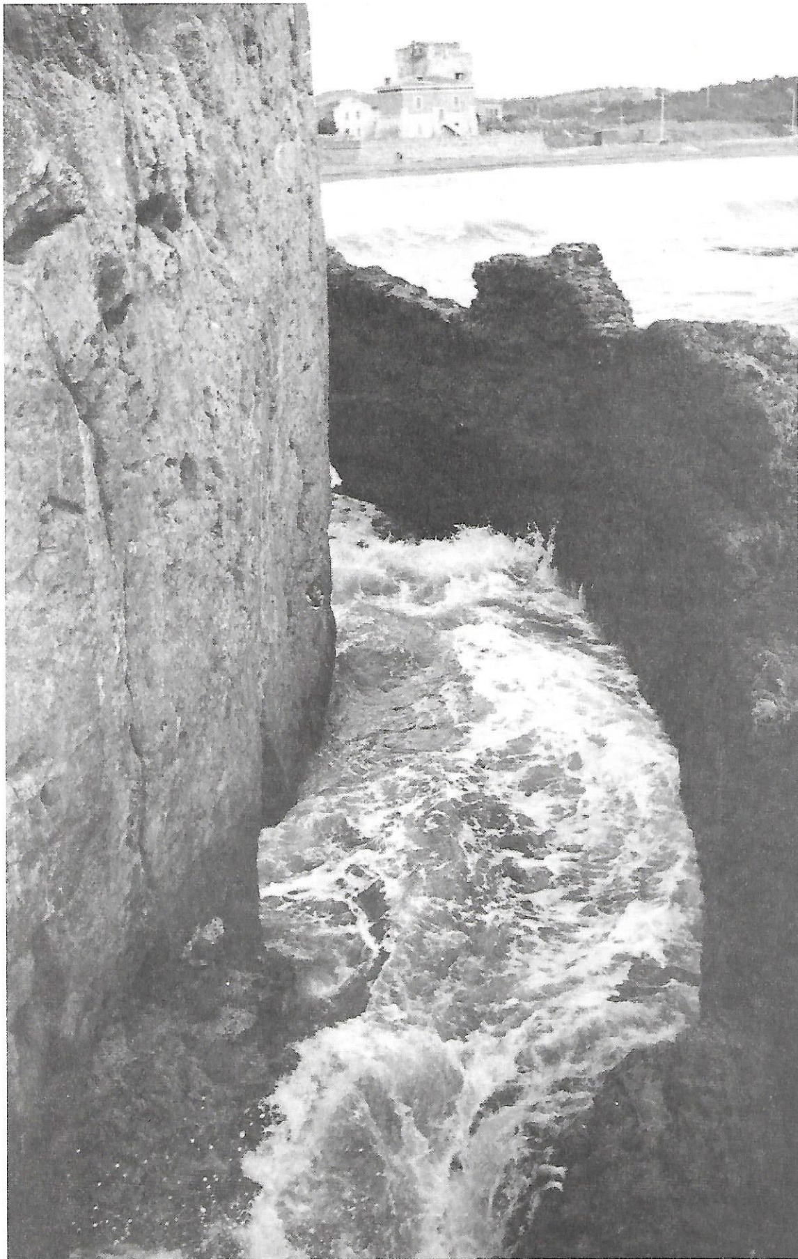
35. Seaward section of Tagliata South, looking north, with entrance of Tagliata Piccola on lower left.
