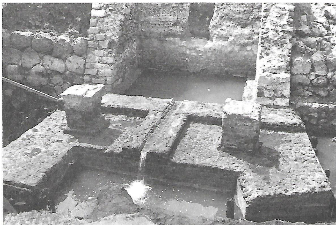
31. Spring House platform, lagoon of Cosa, with collecting tank and water channel. Concrete piers rest on top of platform surrounded by ancient wooden formwork. Retaining Wall P abuts Spring House on northern and southern buttresses.
