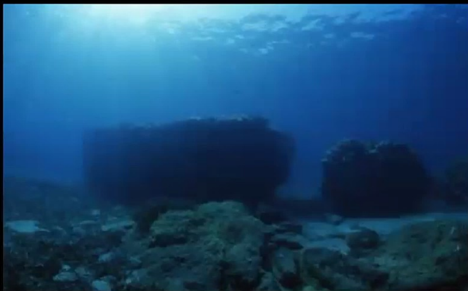
Pier of the harbour
