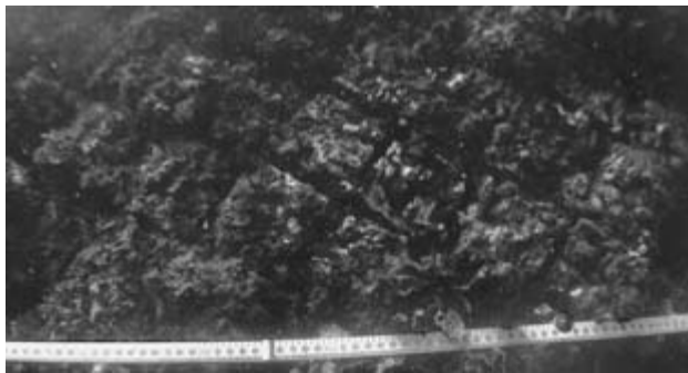
Figure 4. Opus reticulatum at a depth of 6 m on the southern face of a pila at Secca Fumosa. (C. Brandon)
