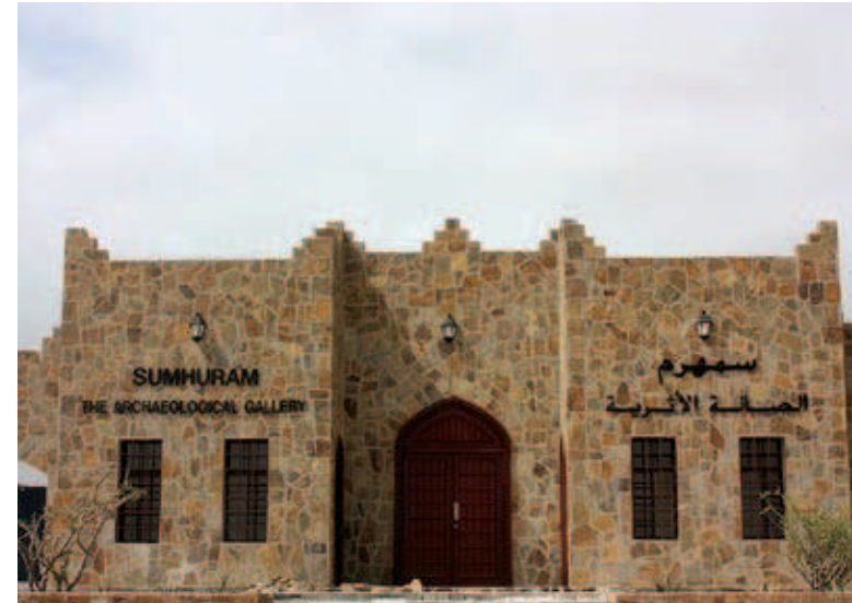
Fig. 1 The new Sumburam Gallery recently inaugurated on the site.
