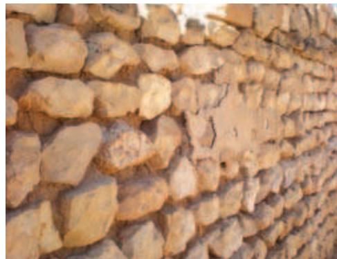
Fig. 5 Example of a wall in Sumburam, made from stone blocks of regular size, arranged in horizontal rows.
