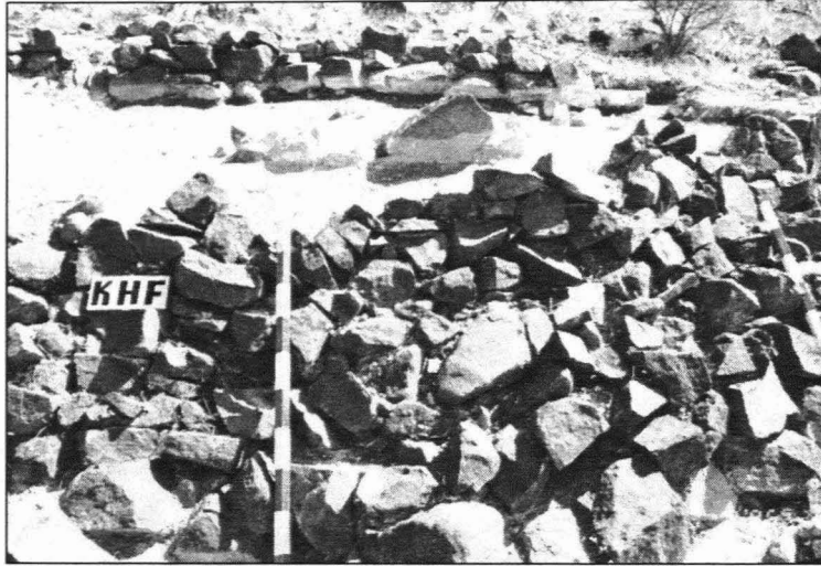
Fig. 26. A view of Building Unit H10 showing the stone façade of the platform and the basin inside room 17.
