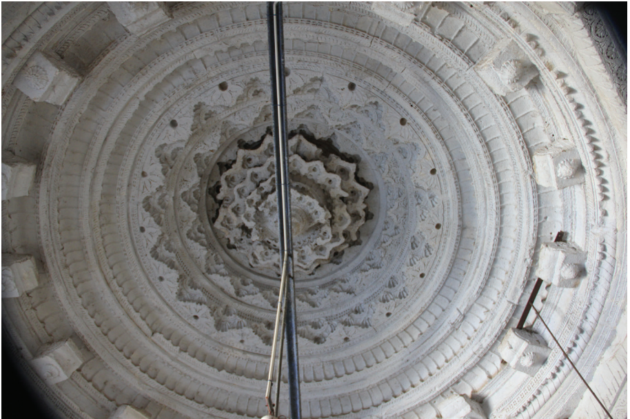
FIGURE 4.10: CEILING OF THE MOSQUE AT MANGROL, GUJARAT
