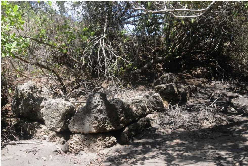
Fig. 4.46 Massive roughly dressed corral blocks forming one of the sea walls currently running along the high water mark.
