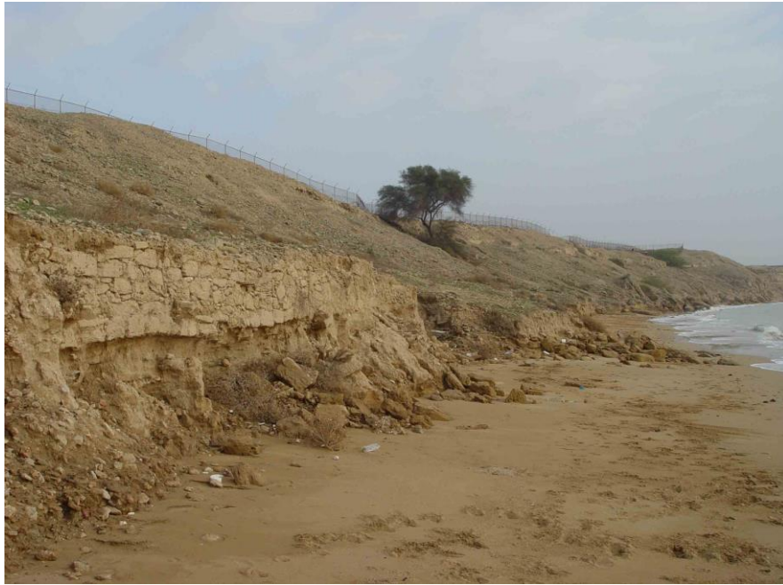
Fig. 4.13 Eroding shoreline section below the southwest defences at Rishahr with traces of a long section of stone wall construction exposed above older occupation deposits.
