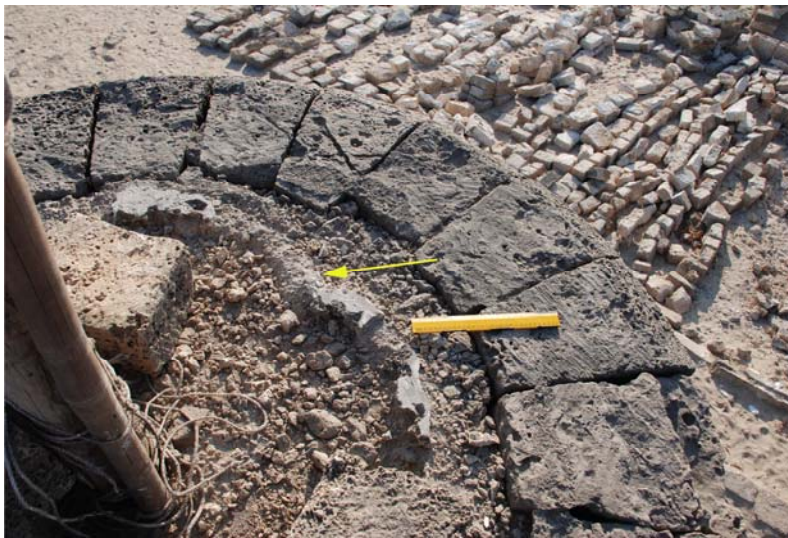
Figure 5. Arrow mark indication some remains of brazier on the top of structure damaged during 1982 cyclone (Photo: A.S. Gaur).
