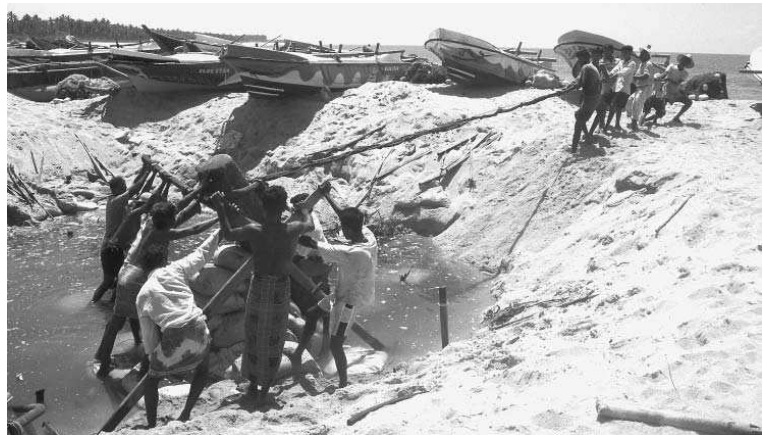
Fig. 224. GODA 5, Re-erecting gneiss pillar 2. A traditional constructing tool, consisting of two right-angled, laced palmwood beams supported the lever.
