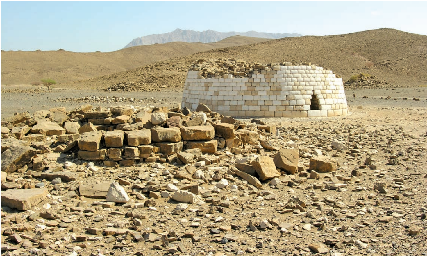
Fig. 9. Bat, tomb 154; the completed work in October, 2008. In the foreground, the remains of the first courses of a tomb of the same construction type as 154.
