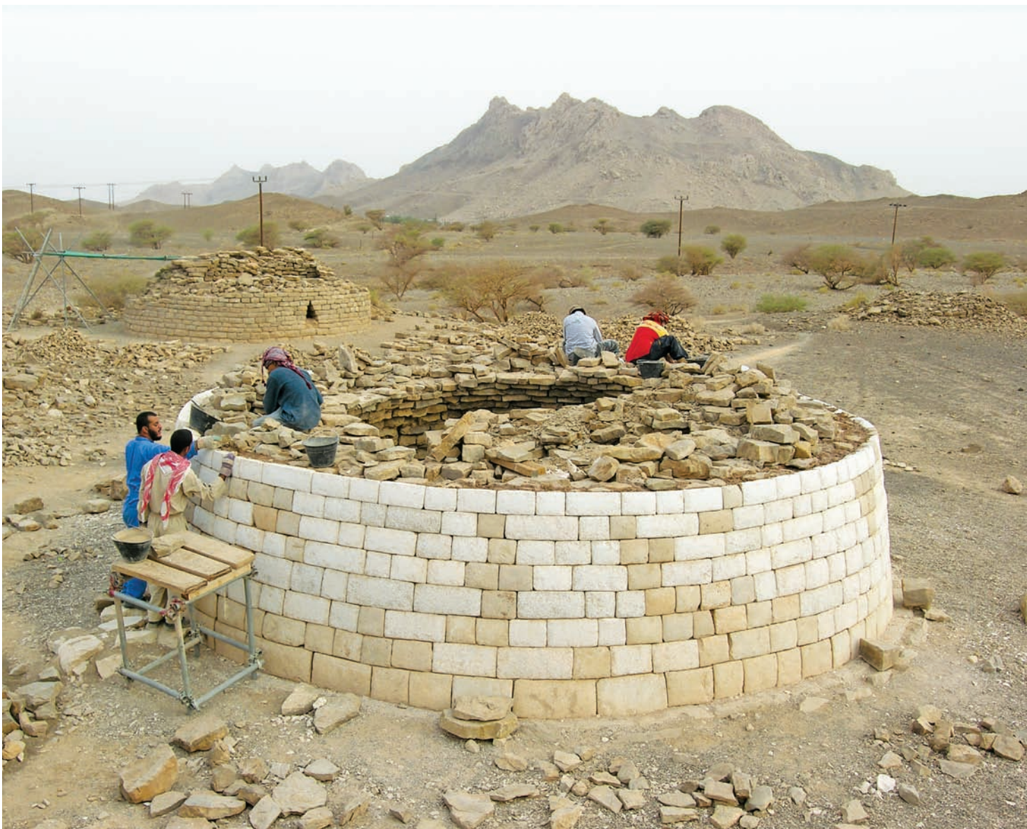
Fig. 8. Bat, tomb 154; completion of the outer layer. The quarries for white limestone are situated in the mountains in the background.
