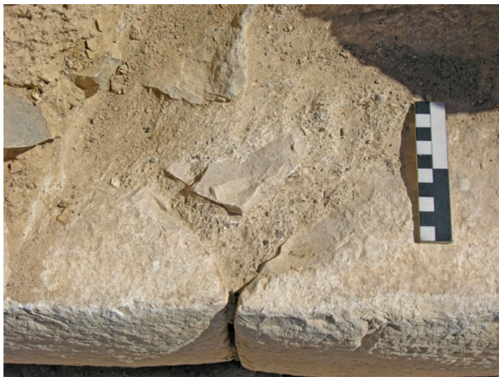
Fig. 4. Bat, tomb 154; the evidence of mortar with quicklime. Scale 10 cm.
