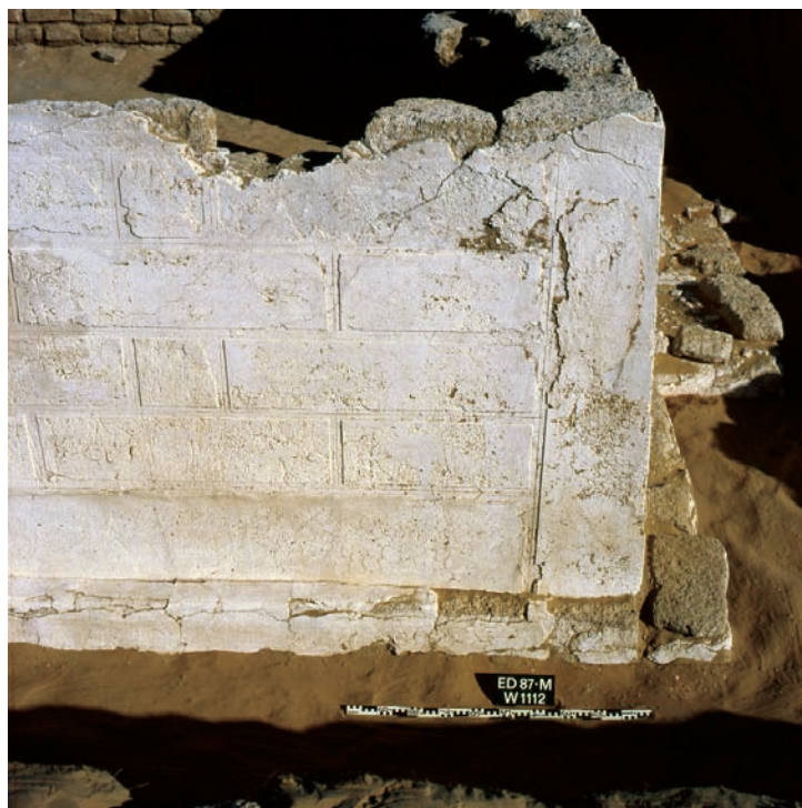
Fig. 6. Detail of plaster decoration on south-eastern wall.
