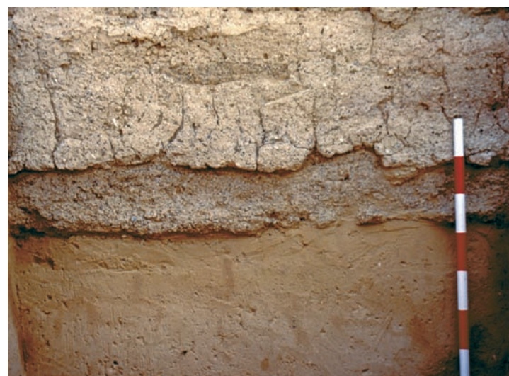
Fig. 2. The houses were built directly on the sand.
