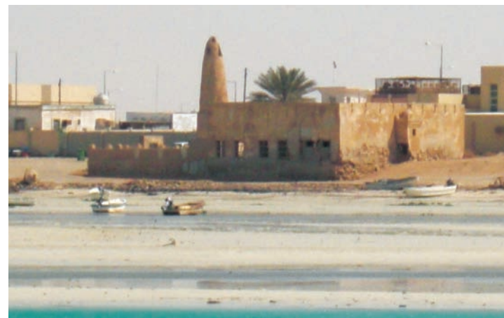
Fig. 5. Ruwais coastal mosque, Qatar. Most coastal settlements had a mosque by the shore for fishermen and travellers. The mosque provided a means of identification and also aided in navigation.
