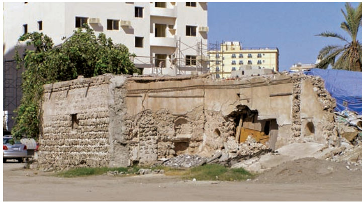
Fig. 6. Ruined coral building on the Sharjah waterfront. Preliminary examination identified at least three types of coral in this building.
