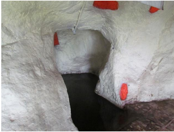
Figure 8: Unfinished inner chamber filled with water.
