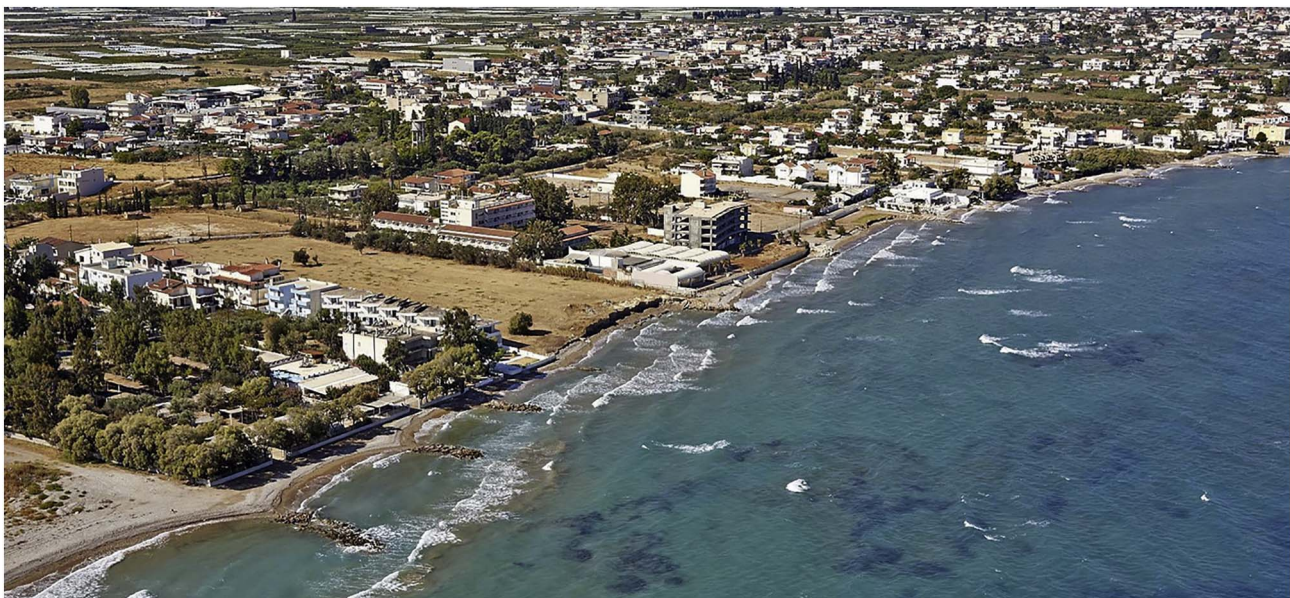
Fig. 6. Aerial view of the extensive coastal protection works along 4 km of coastline, 1.3 km east of Lechaion up to Assos. (Image from https://www.tripinview.com/en/presentation?layer=detailed&datasetId=58007&id=39026 , 2014 Geotag Aeroview.)
