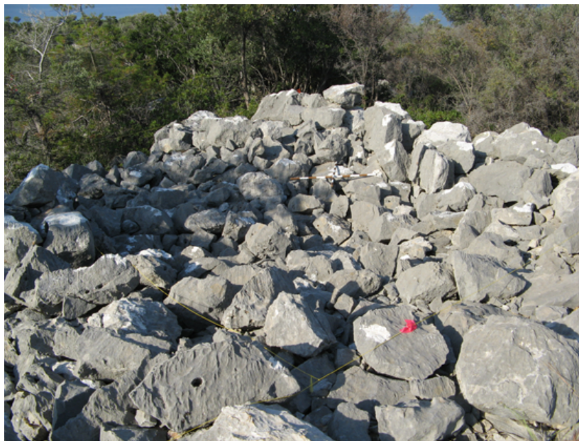
Figure 24. Building 4-VI, room 6: overview showing collapsed rubble
