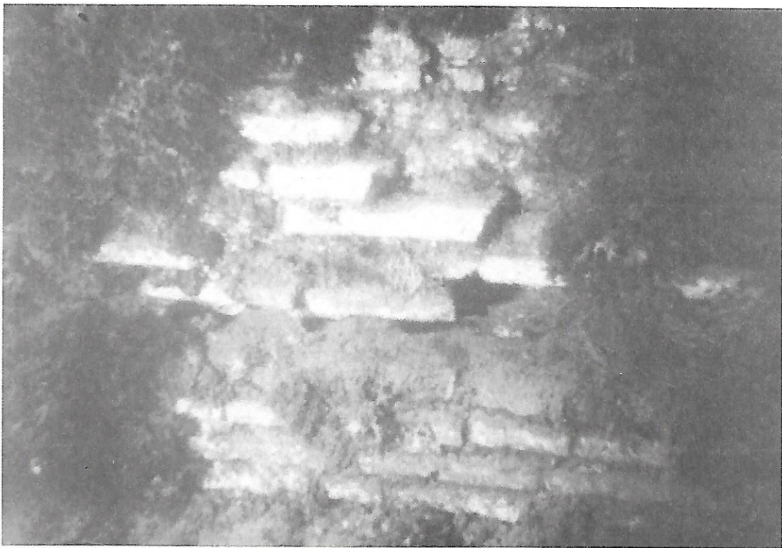
Fig. 7. Submerged roman brickwall.
