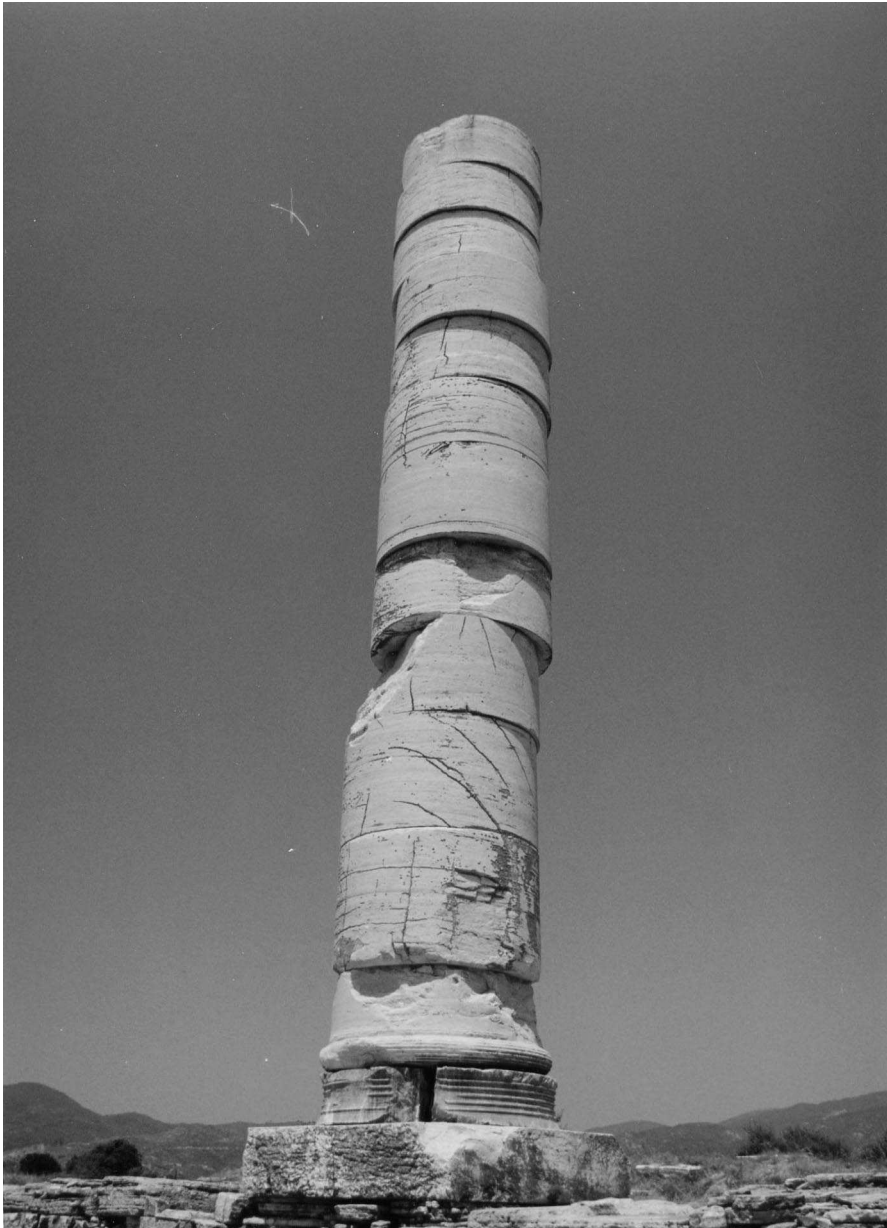
Fig. 11. The only surviving column of the Heraion temple, near Pythagorion, constructed in circa 530 BC. Displacement of the drums testifies to rocking caused by high seismic accelerations (see Stiros, 1996), similar to those expected to have been produced by earthquakes responsible for the coastal uplift of the Karlovasi area.
