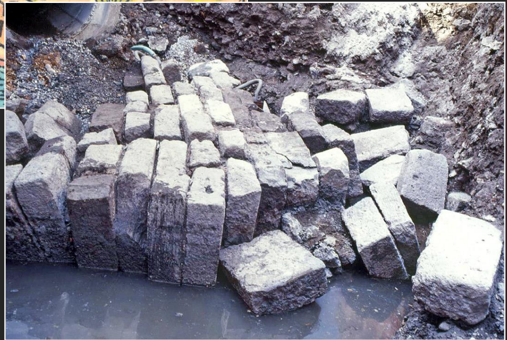
Ashlar blocks from the deck of the large bridge.
