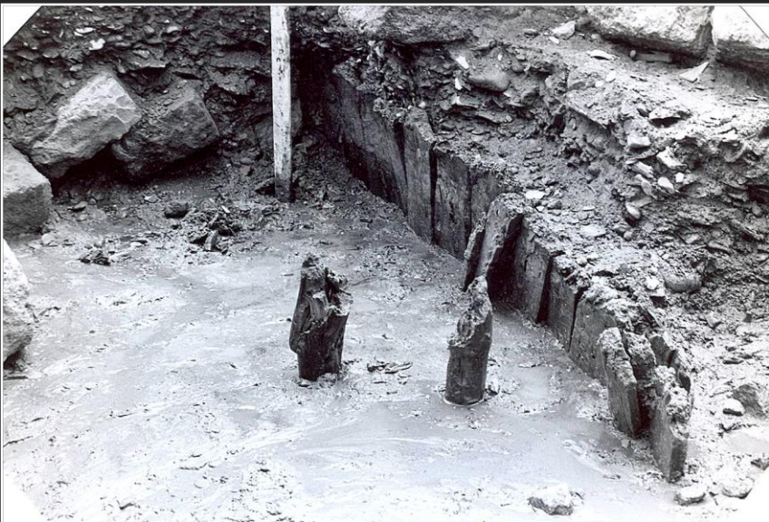
Wooden piles and frames to strengthen the foundation of the jetty structure in the sandy saturated bottom.
