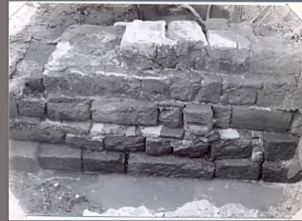
Later repairs where hydraulic mortar and column drums were used
