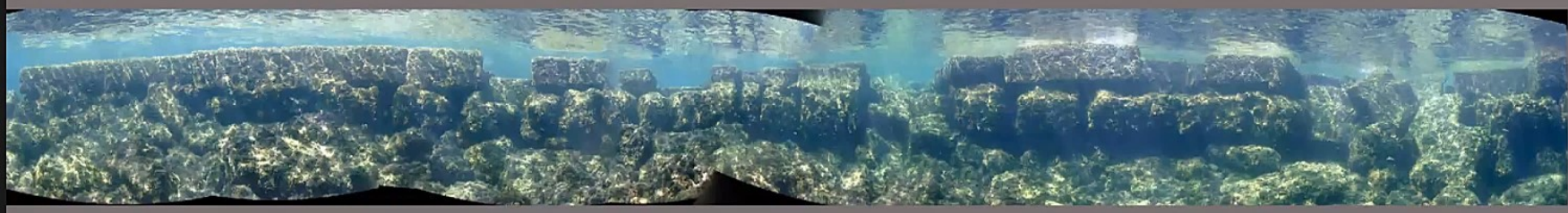
Underwater view of the rectangular transverse opening - 'channels' at the southeastern breakwater of the North harbor of Mytilene
