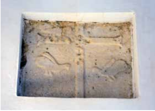
3b.2. Chora, Catholic church of St Andrew, closure slab with decoration common on reliefs of the second phase of the basilica at Palaiopolis.
