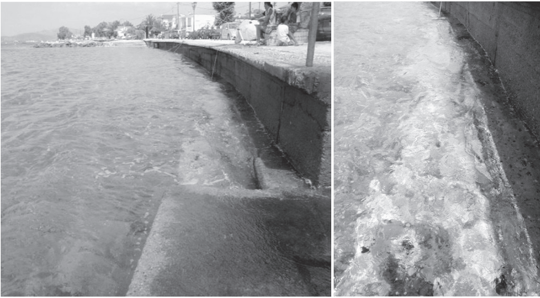
Fig. 5. Central quay construction at Platanidia. (Photos: A. Ginalis)
