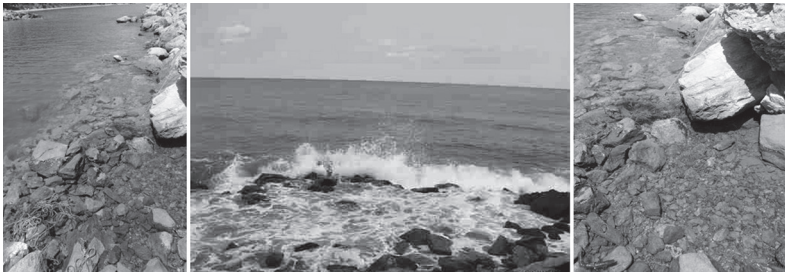
Fig. 17. The northern breakwater of Koutsoupia. (Photos: A. Ginalis)
