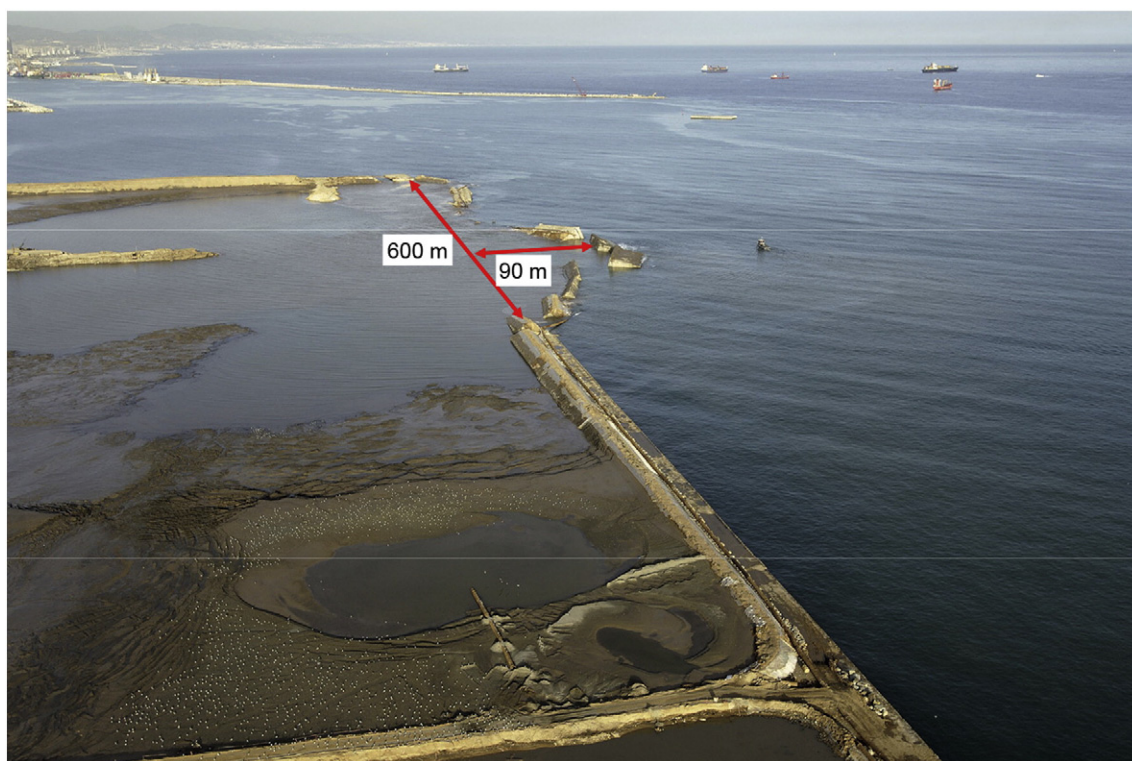
Fig. 7. Failure of the Prat Quay, Barcelona harbor in 2007 due to static liquefaction, which produced lateral offsets of the order of 90 m (after Gens, 2015). Such static offsets highlight the potential of dynamic liquefaction to excessively amplify seismic strike-slip motions.
