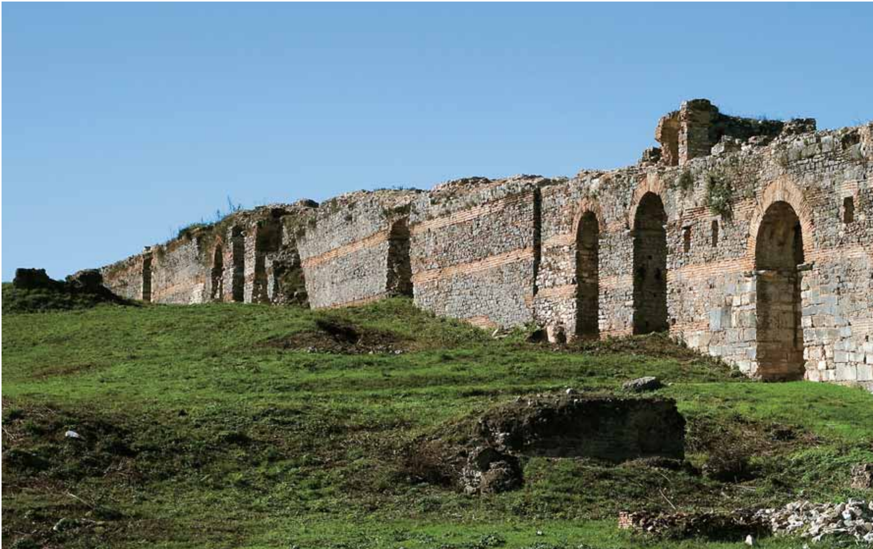
Fig. 126 | Nikopolis, west part of the Early Christian walls.
