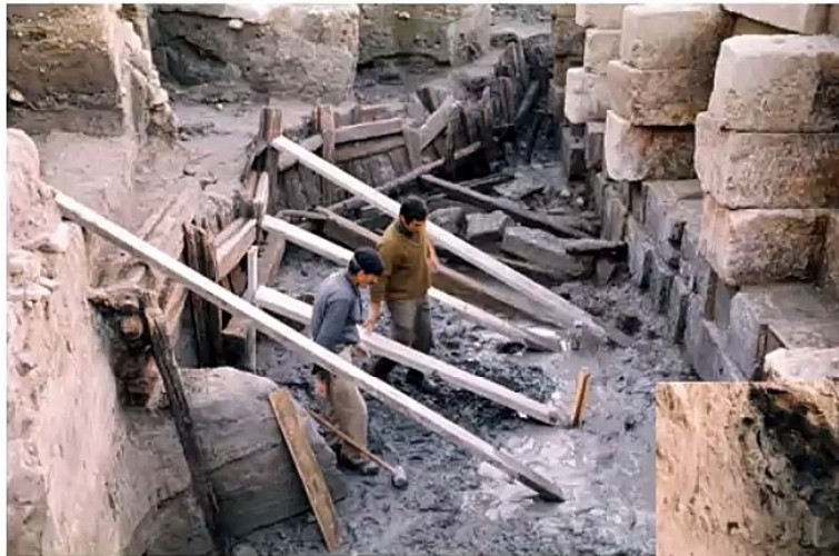
Cofferdam system of the freshwater basin (© Antoine Chenet, CNRS-CCJ, 1972)
