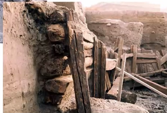
Cofferdam system of the freshwater basin (© Antoine Chenet, CNRS-CCJ, 1972)
