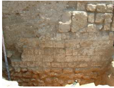
Fig.7. The Western wall of the building „A”
