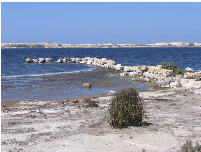
Fig. 7 – The eastern quay of a box-shaped harbour that was recorded on the southern shore of the lake. This harbour appears to have gone through several phases of use, however, its original date is not established (Photo by E. Khalil).
