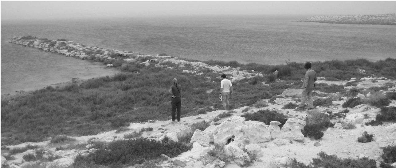
Fig. 4: The middle quay of the harbour of Marea (photo by: E. Khalil).
