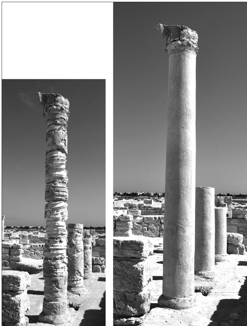
Fig. 5. House H10a. Damaged columns before conservation in 2012 (left) and after (Photos R. Czerner)
