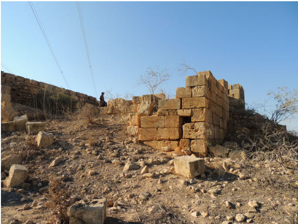
Figure 40. The north-west tower of the gasr (KHM 105), showing the different quality of the masonry, ashlar blocks still in situ and other reused ashlar blocks, on the west face. Photo: Archaeological Mission Roma Tre University. (Colour online.)
