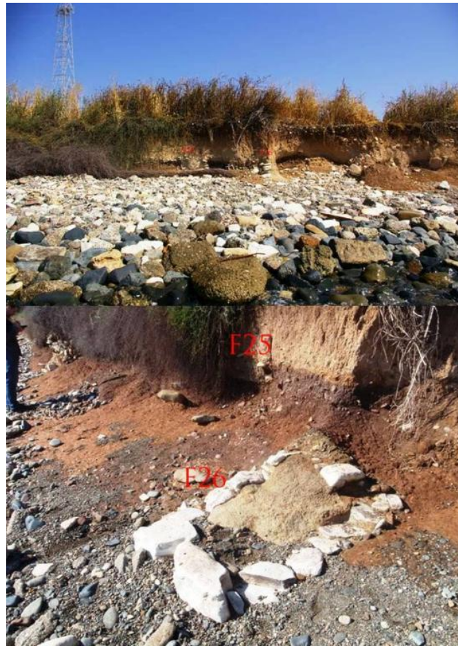
Fig. 1.12 Tochni-Lakkia, example of diachronically eroding clay-filled, stone-lined feature (June 2011, June 2013 – D. Sewell).
