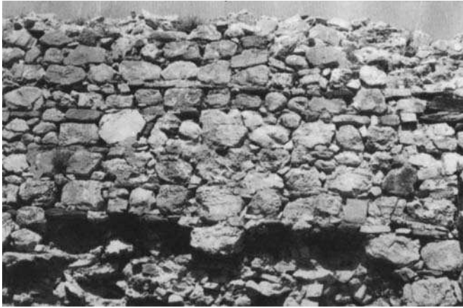
Figure 13 Roman warehouse: dolomite exterior facing
