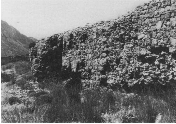
Figure 15 Roman warehouse: east face from north; detail of buttressing
