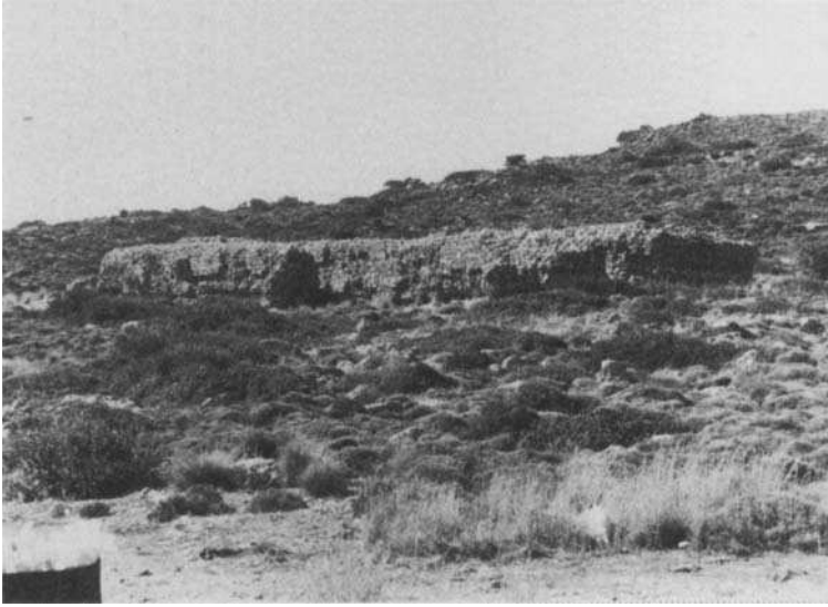
Figure 17 Roman warehouse: interior from south
