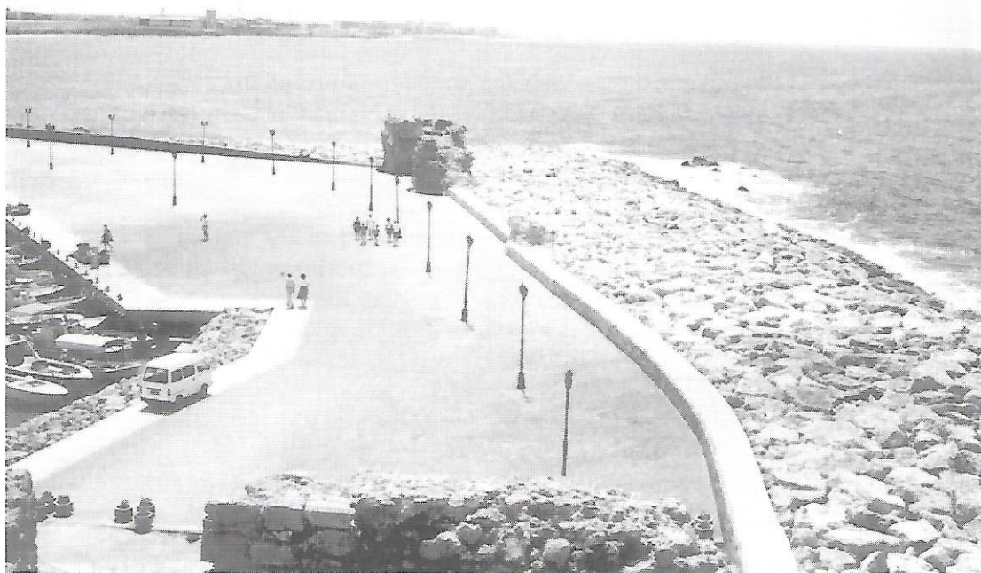
Figure 8. Renovations to the western breakwater at Paphos in the 1980s, namely, the addition of a ca. 23 m. wide rubble baffle, allowed the port authorities to remove a seawall that had once formed the main defensive line against storms. Ruins in the sea south of the remains of the Frankish Fort mark the line of the ancient spur. Photograph by R. L. Hohlfelder (looking E)
