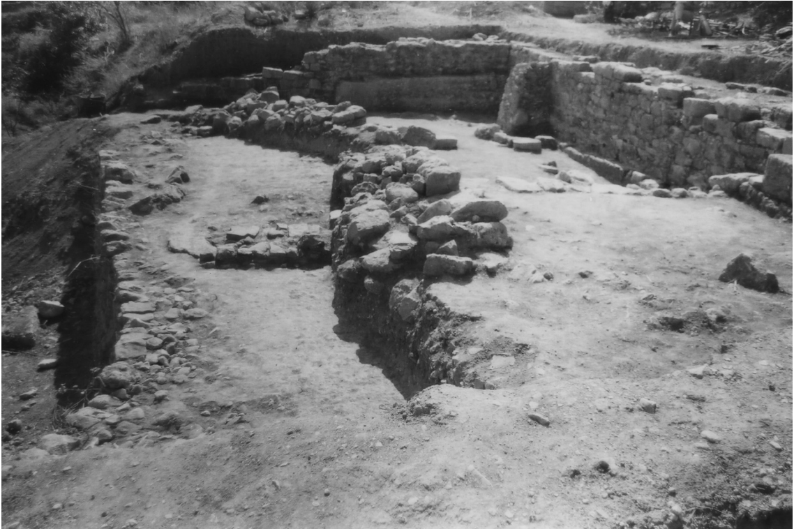
FIG. 15 – VOUGIOUKALAKIS PLOT: TRENCH 5, LOCATION OF PIT WITH GEOMETRIC OSTRAKA, FROM EAST OF WALL 2.
