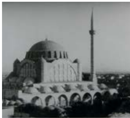
Image 5. Mihrimah Mosque, a work of Architect Sinan
