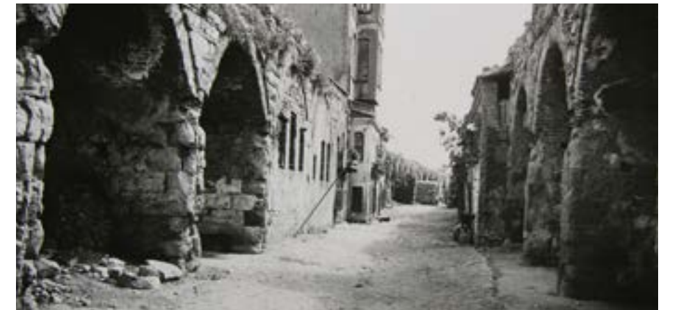
Image 16. Dilapidated structures of Sultan Ahmet Arasta
