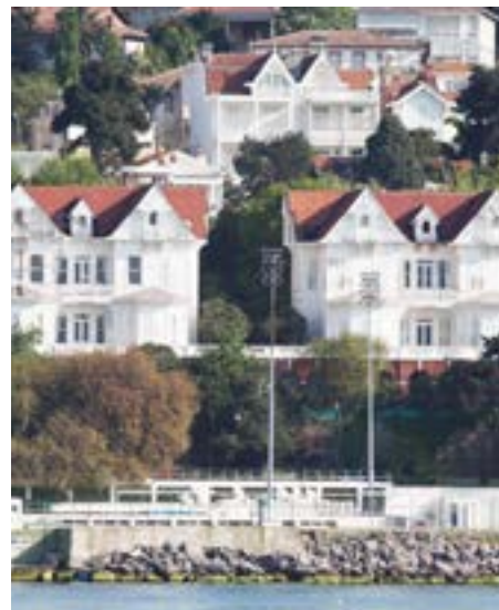
Image 15. Island skyline formed by buildings positioned in harmony with the inclinations of the topography
