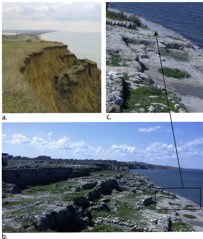
Fig. 7. Cliff erosion of the Taman Peninsula on the present shores of the Azov Sea (a) from Fouache et al. (2012) and in the Taman Gulf at the Greek settlement of Hermonassa (present Taman) which is rapidly being lost to the sea (b). Zoom on engineering structures to control erosion at Hermonassa (c).
