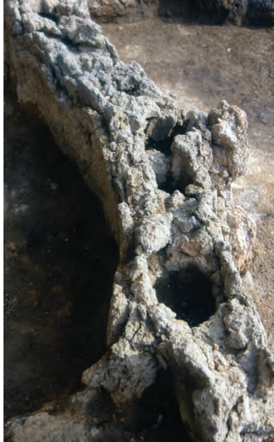
Fig. 147 - Aşağı Pınar, a detail from the wall construction of Layer 6.
