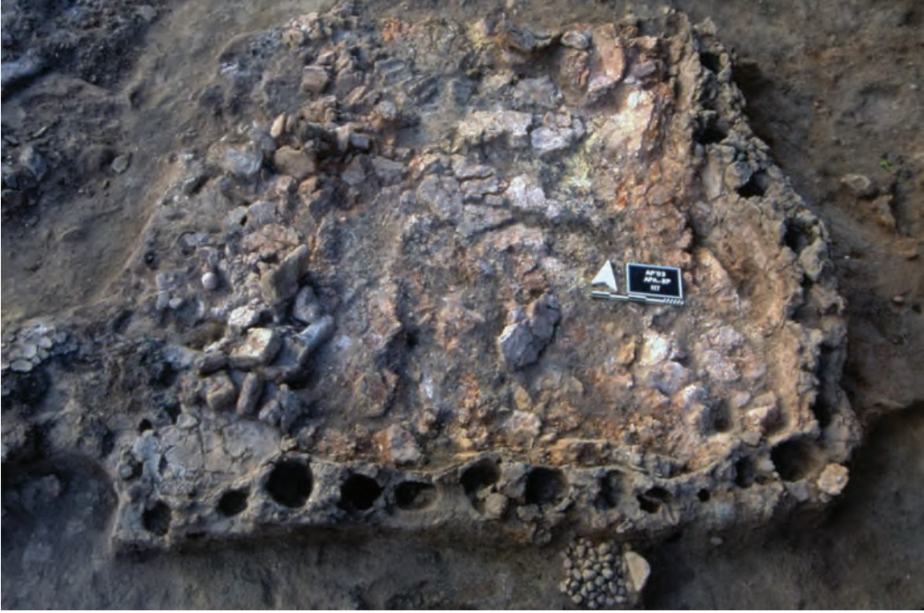
Fig. 146 - Aşağı Pınar, a detail from one of the rooms of Layer 6 building complex, showing the wall construction system.
