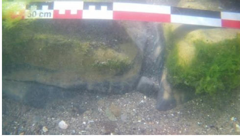
Fig. 15: Detail of Second Set in Front of Modern Concrete Set
